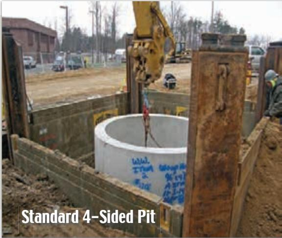
Individual Slide Rail components offer the option of using lighter equipment when installing the system. The cost of rental and installation of the system is approximately 50% of steel sheeting.
