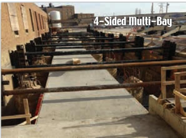
This configuration is ideal when installing next to existing utilities and structures. Longer pipe may be installed by raising or removing the parallel beam spreader assembly.
