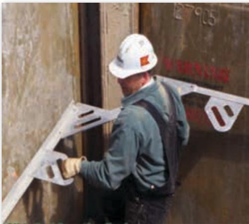
Squaring the system is critical to the ease of the dig and push process. The Squaring Tool is a spacing template that makes it easy to assure that the system is square and plumb.
