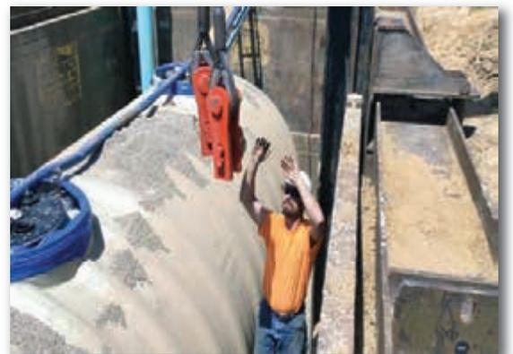
Pull Bracket-Removal Shackles are uniquely designed to quickly and easily pull Slide Rail panels from compacted soil without damaging the panels or other equipment.
