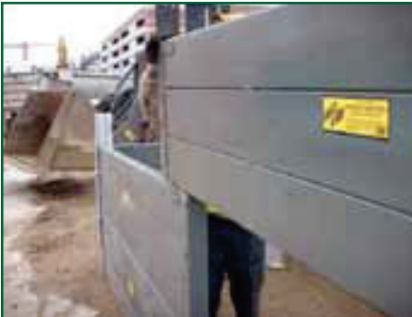
3. Panels stacked to desired height
