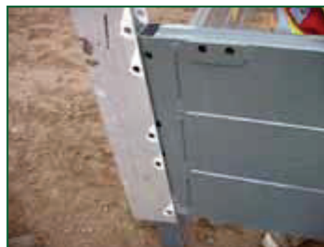
2. End panels set into corner end
