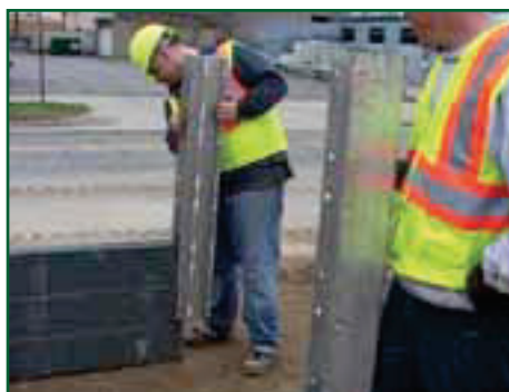
1. Corner end posts pinned on panels
